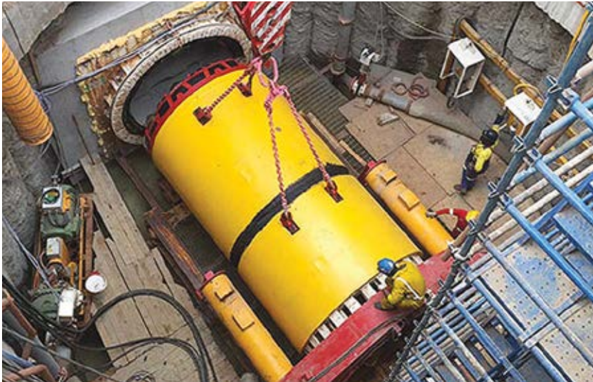
Pipe Jacking Method
